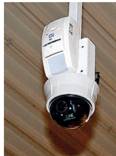
Foto's: Expertise &amp; Security Consultants
